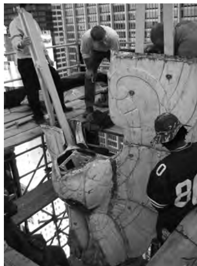
A Beyond roofing, copper is also used for ornamentation. Restoration of this copper eagle atop a 1929 high-rise involved off-site and on-site repair, cleaning, and reconstruction.
